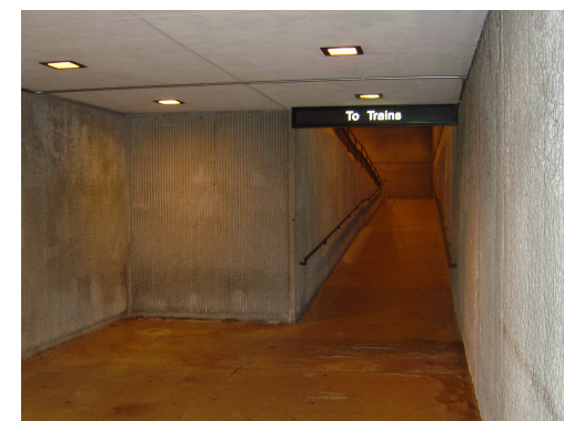
Station house interior
