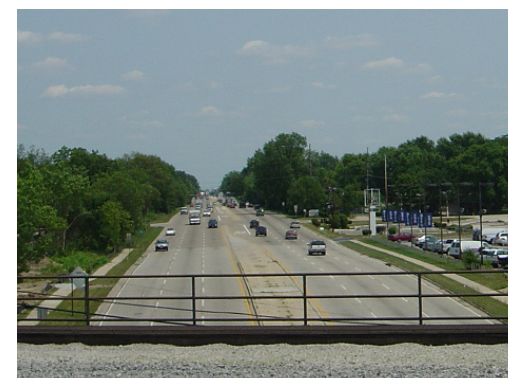
211th Street Metra Station platform (looking east)
