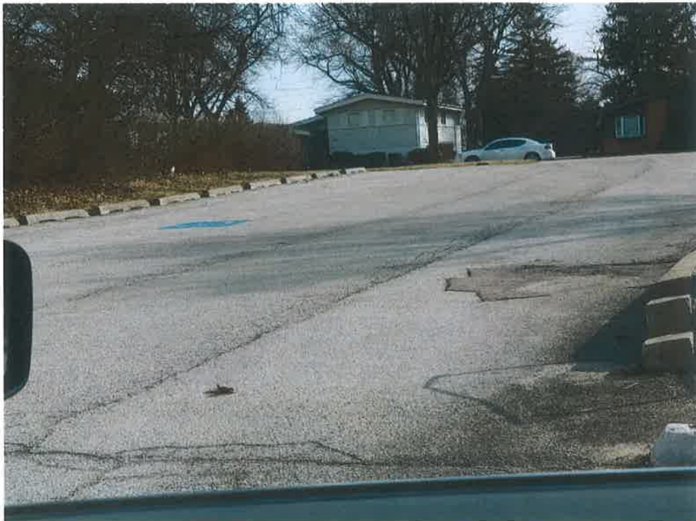
Parking area on Northeast side of building
