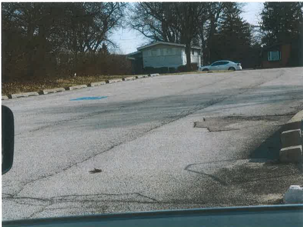
Parking area on Northeast side of building
