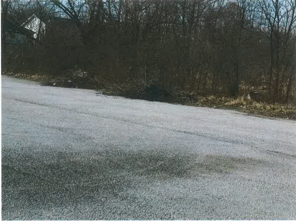
Landscape debris on edge of parking area
